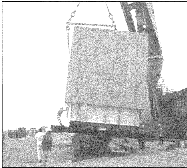
Figure 6.1 – Trailer of insufficient capacity used for cargo discharge
